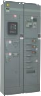
Figure 38: Low voltage motor control center (floor-mounted).
