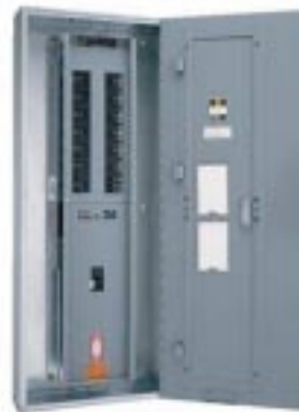
Figure 23: Panelboard (surface wall-mounted).
